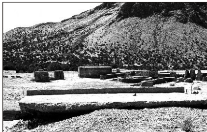
Remnants of the Graphic Mill. The old concrete structures once supported the ball mills, crushers, and other heavy machinery for the mill.
